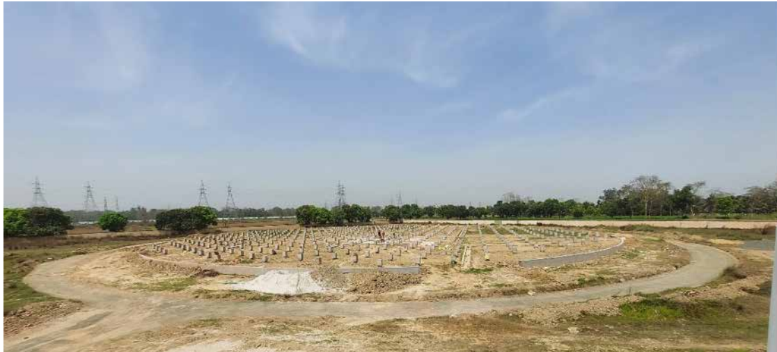
Fig. 3.78: Radar area with antenna pedestals, cable trench, guard wall and perimeter road
